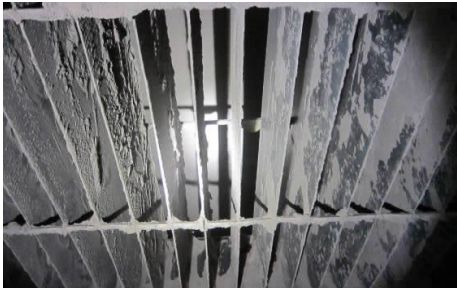
图 4 第 1 层催化剂上后部整流格栅( 灰多) Fig.4 Rear rectifier grid on the first-layer catalyst( much ash)
