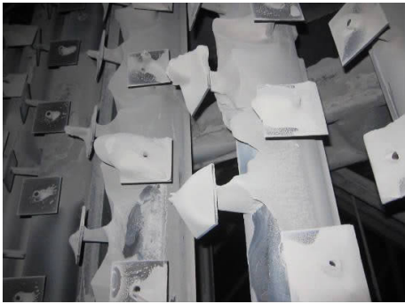
图 2 喷氨格栅上部( 积灰多,未见磨损) Fig.2 The upper part of the ammonia-injecting grid( with accumulated ash and no wear)
