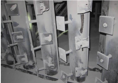
图 1 喷氨格栅下部( 积灰少,局部有磨损) Fig.1 The lower part of the ammonia-injecting grid( with little ash and local wear)
