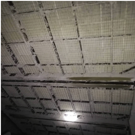
图 6 靠后烟道脱硝催化剂底部正常无磨损 Fig. 6 No abrasion at the bottom of denitration catalyst in rear flue duct
